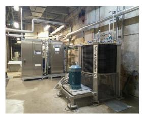
• **Technology uniqueness and comparison vs state-of-the-art**: Valmet Ultrafiltration Tissue is the first new designed cross rotational ultrafiltration system for Tissue mills white water recycling and purification. State of the art nowadays is the warm fresh water for the critical consumption points.
