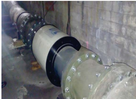
Installed at AM
